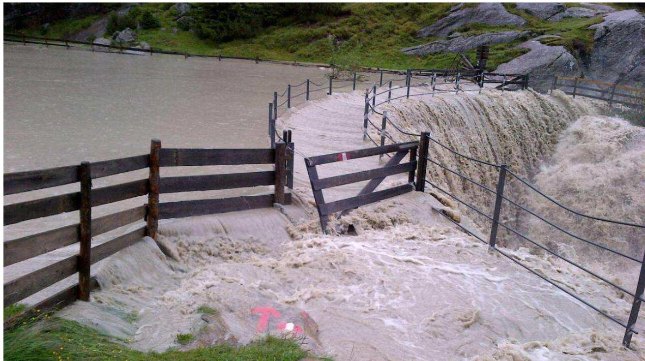
**Figure 1.** A flash flood occurred August 13<sup>th</sup>, 2014 and the water masses overtopped the Aglsboden/Pian dell'Accl Dam in the watershed which drains the Malavalle – Übeltalferner glacier (picture: Volunteer Fire Department Ridnaun/Ridanna).
